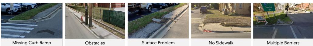
Figure 1. Examples of sidewalk accessibility barriers. The last sub-figure shows multiple barriers present together: missing ramp, no sidewalk, and uneven surface. Images from Project Sidewalk [78].
